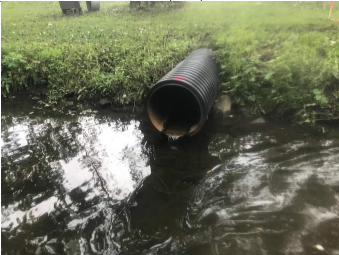
Photograph No. 44 STA 30+75 18" CPP
