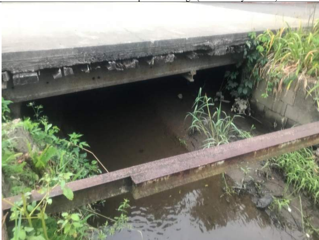
Photograph No. 18 STA 14+00 Upstream photo of bridge (16ft wide by 34" tall)
