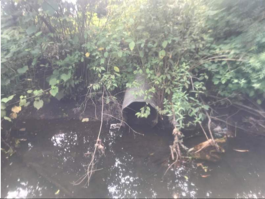
Photograph No. 9 STA 10+50 18" CMP on East side of creek
