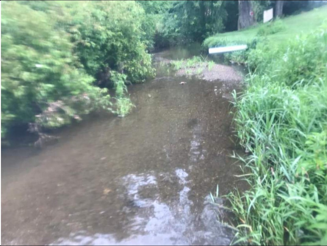
Photograph No. 47 STA 33+75 Downstream photo
