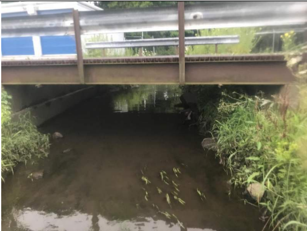
Photograph No. 25 STA 17+50 Upstream photo of bridge (12.5 ft wide)
