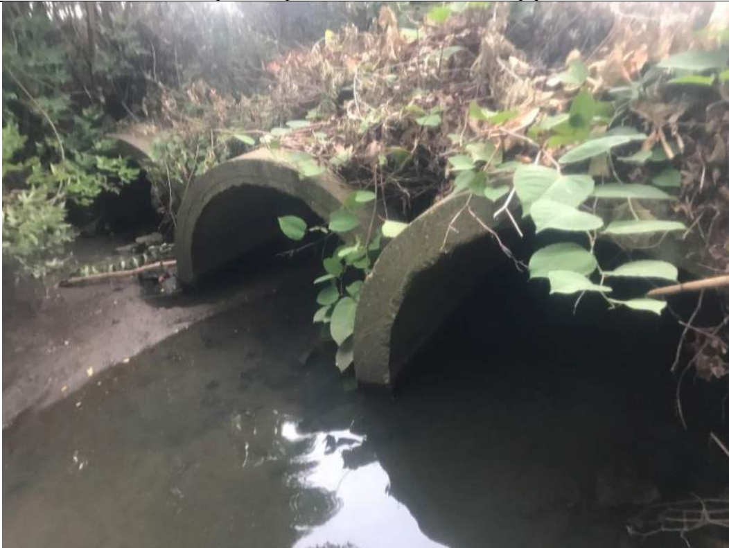
Photograph No. 14 STA 13+00 Downstream photo: 3 RCPs
