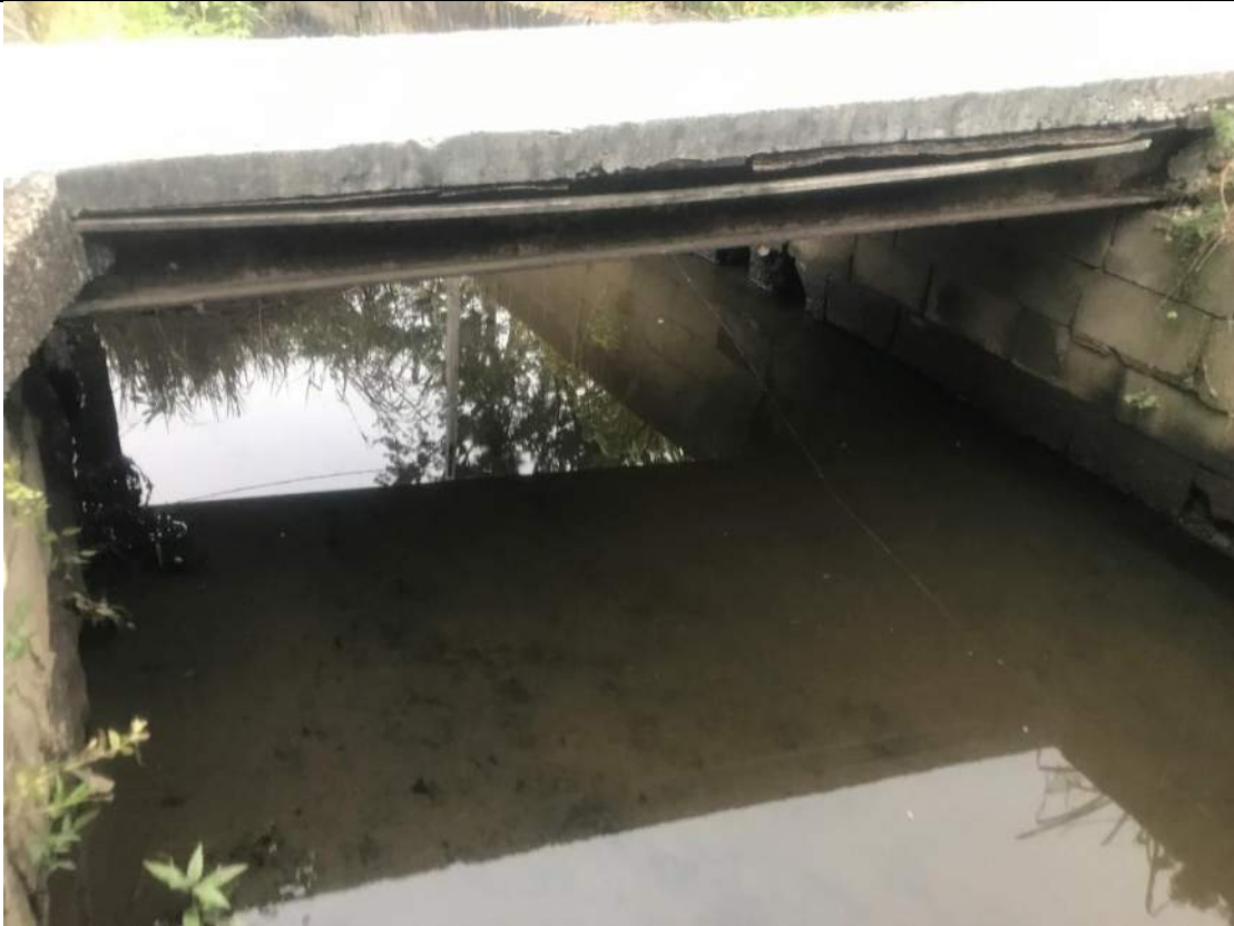
Photograph No. 20 STA 14+75 Upstream photo of bridge
