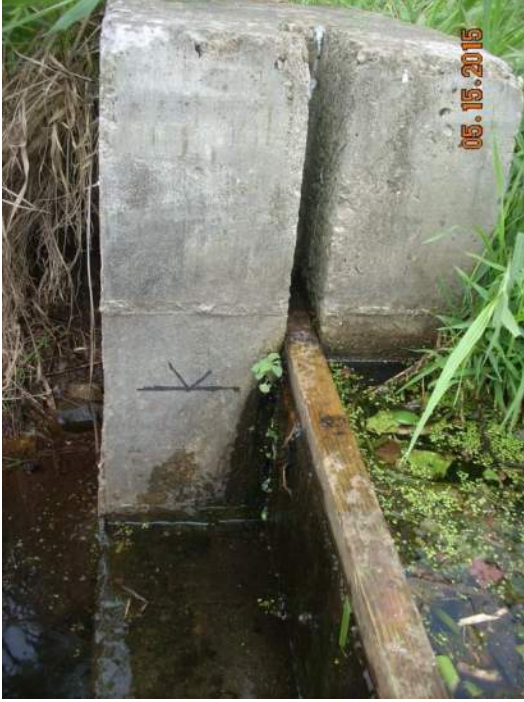
Maximum Lake Elevation marked on east abutment
