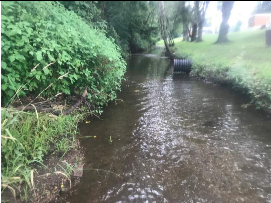
Photograph No. 42 STA 30+50 Downstream photo
