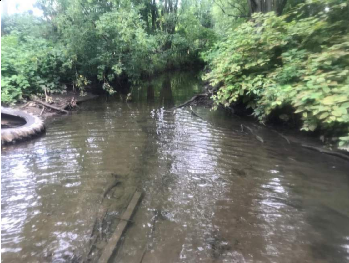
Photograph No. 61 STA 46+00 Downstream photo
