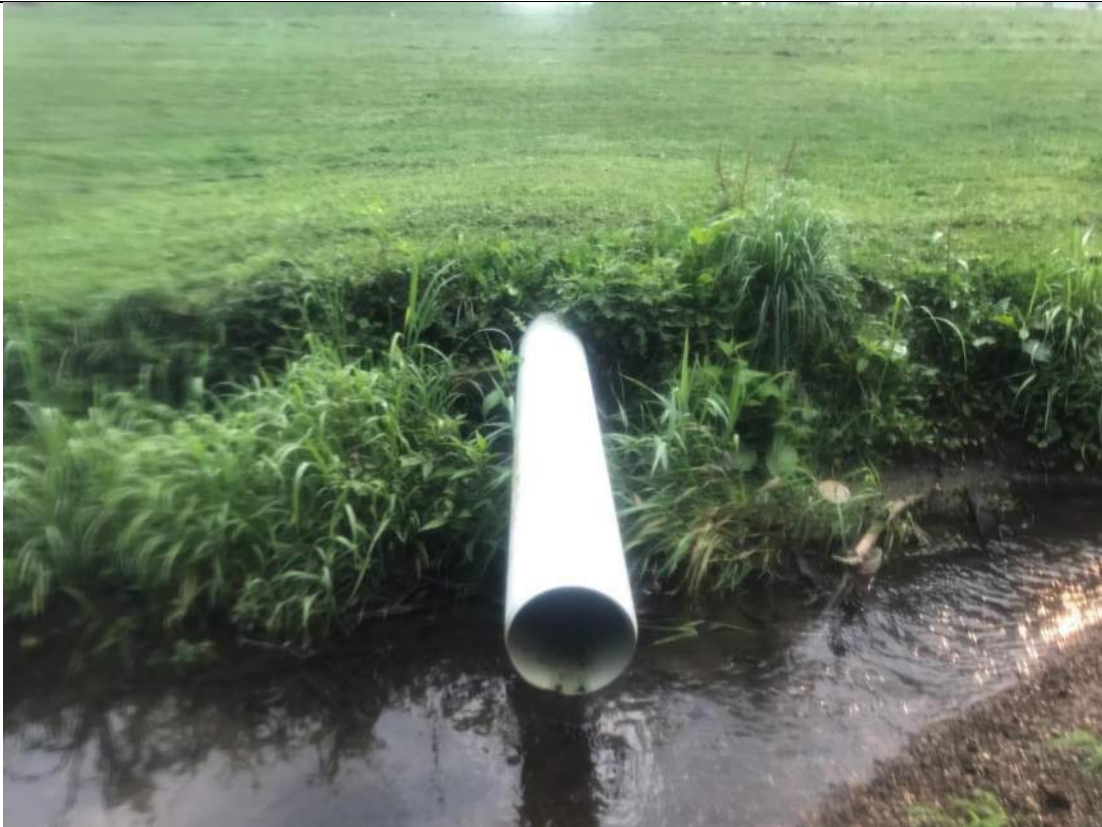
Photograph No. 50 STA 34+00 8" PVC on East side of creek
