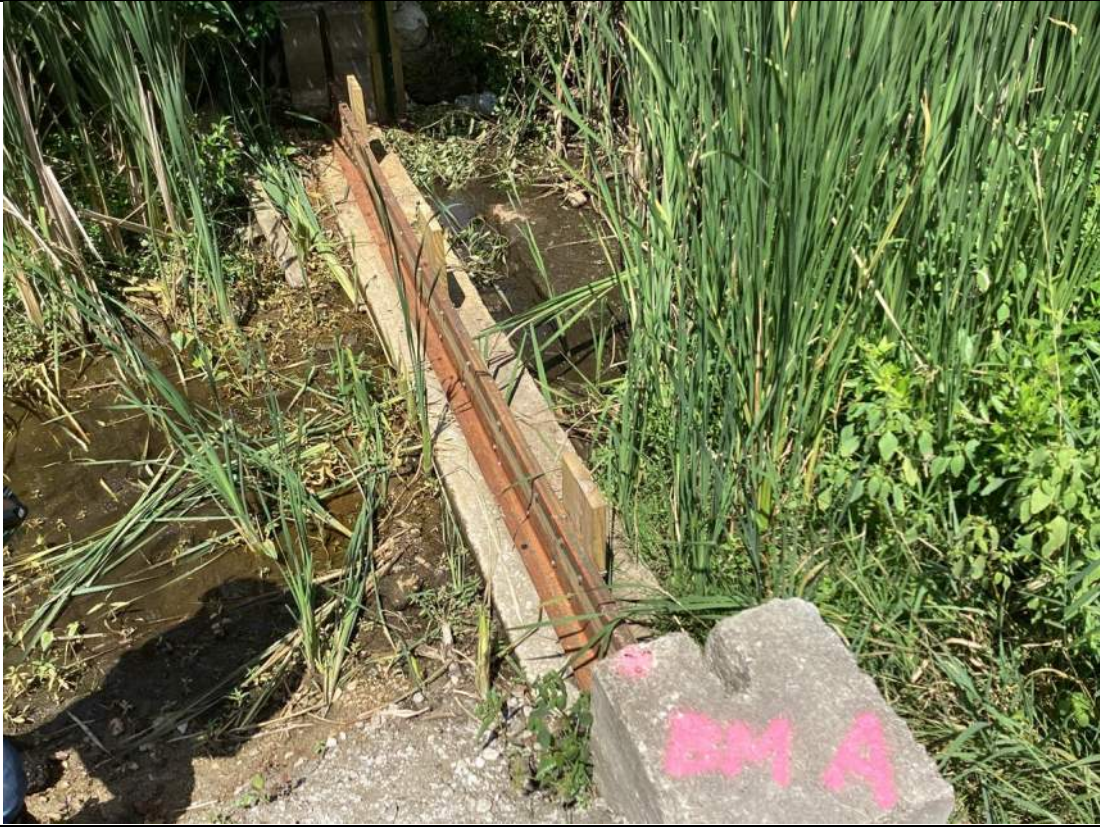
Photograph No. 9 Water Control Structure
