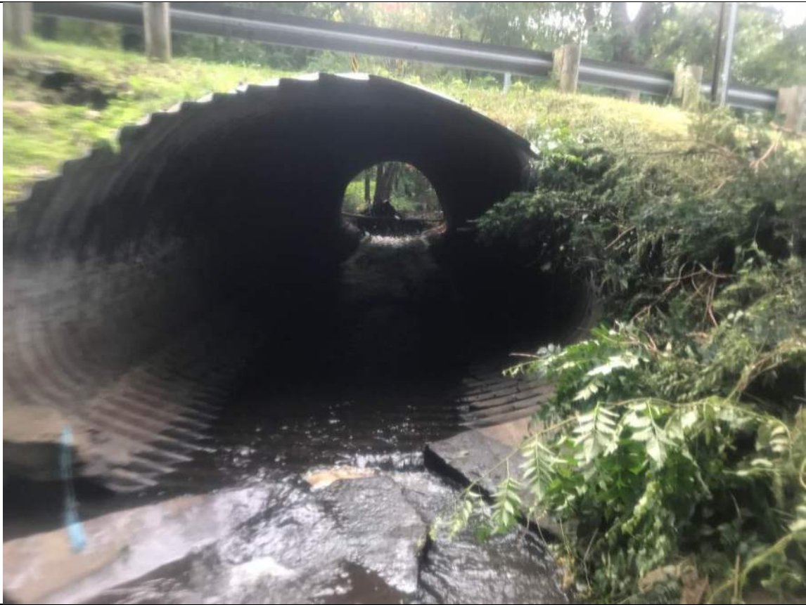
Photograph No. 69 STA 51+50 Upstream photo (11.5ft wide by 7'4" tall road crossing)
