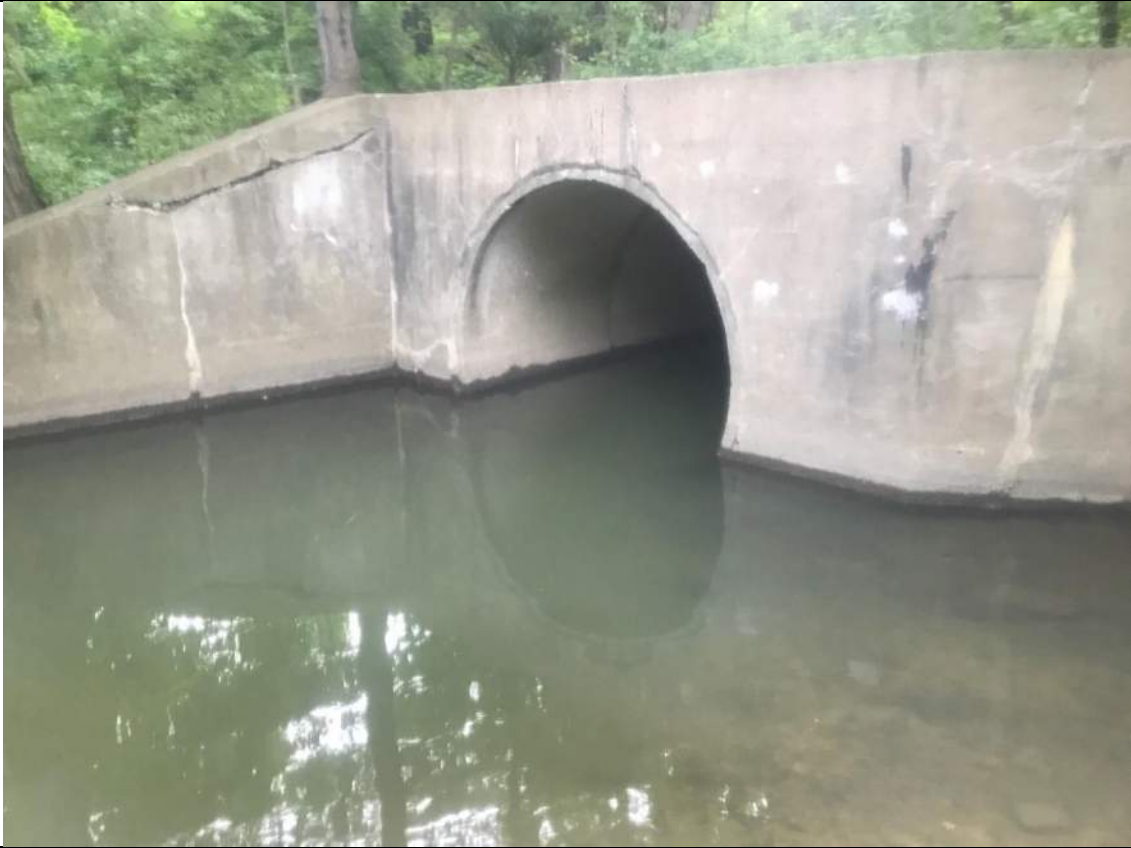
Photograph No. 65 STA 48+50 72" RCP on East side of creek
