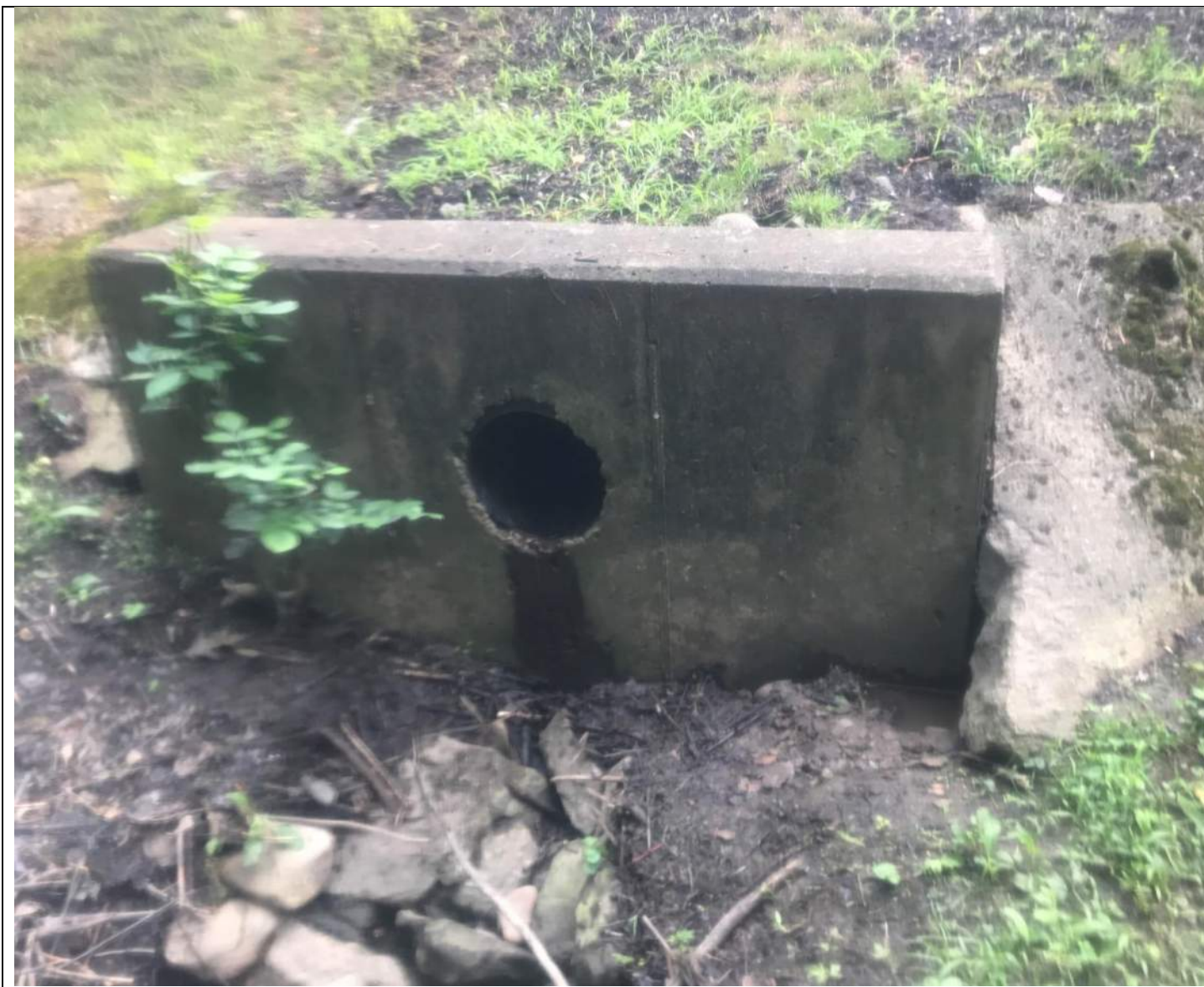
Photograph No. 75 STA 56+00 12" metal pipe just past county line
