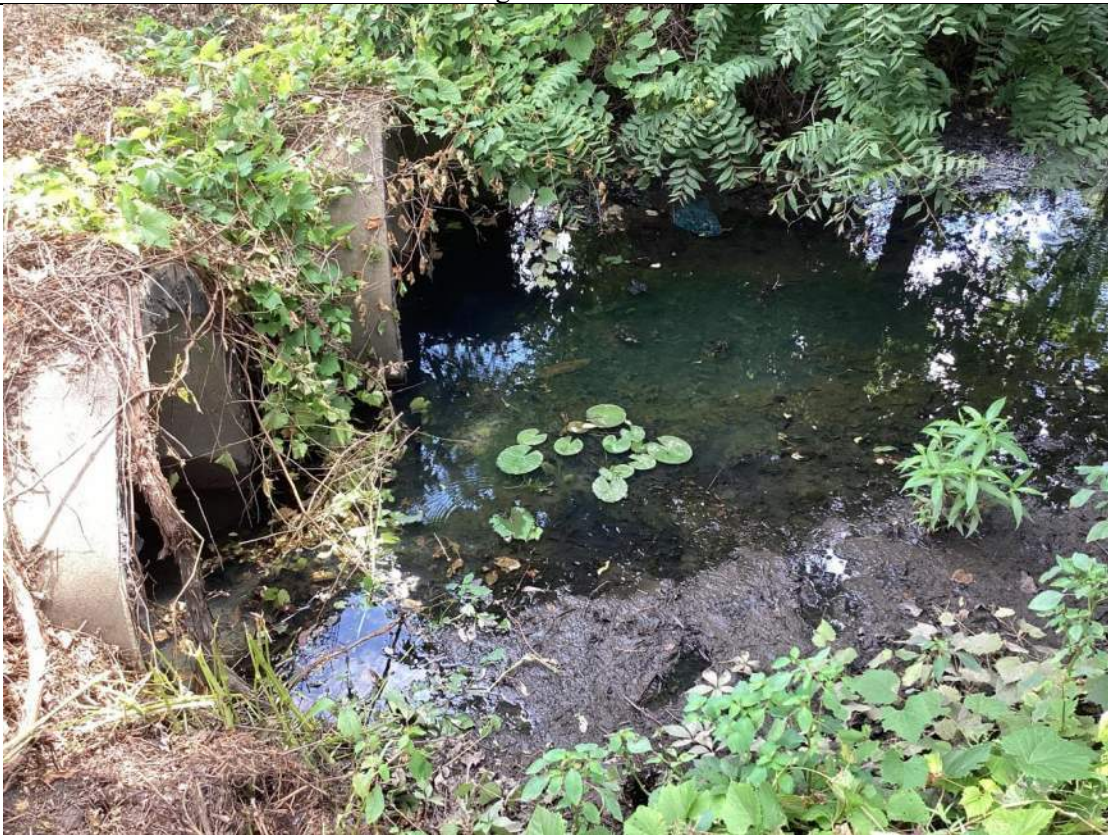
Photograph No. 2 Culverts along Main Channel Stream
