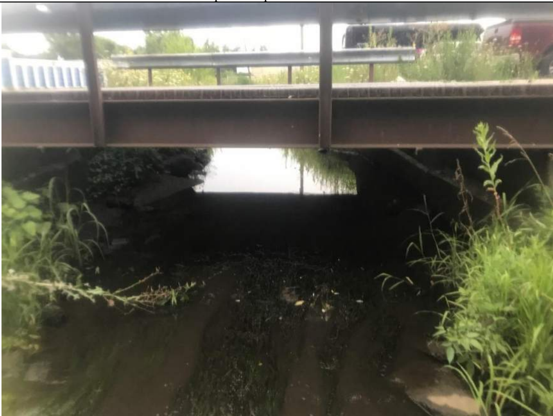
Photograph No. 24 STA 17+50 Downstream photo of bridge (12.5 ft wide)
