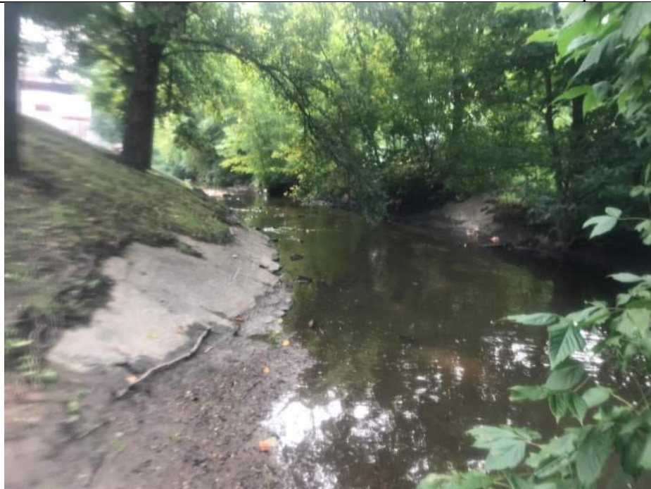
Photograph No. 74 STA 56+00 Upstream photo
