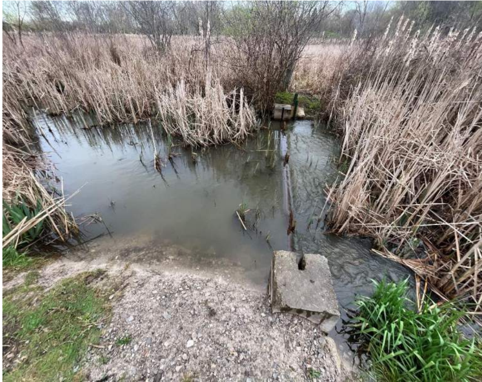
Photo 7 – View of Springfield Lake Outlet stream and structure.
