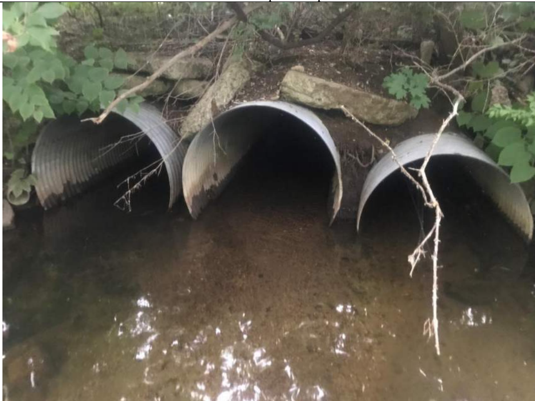
Photograph No. 16 STA 13+00 3 pipes
