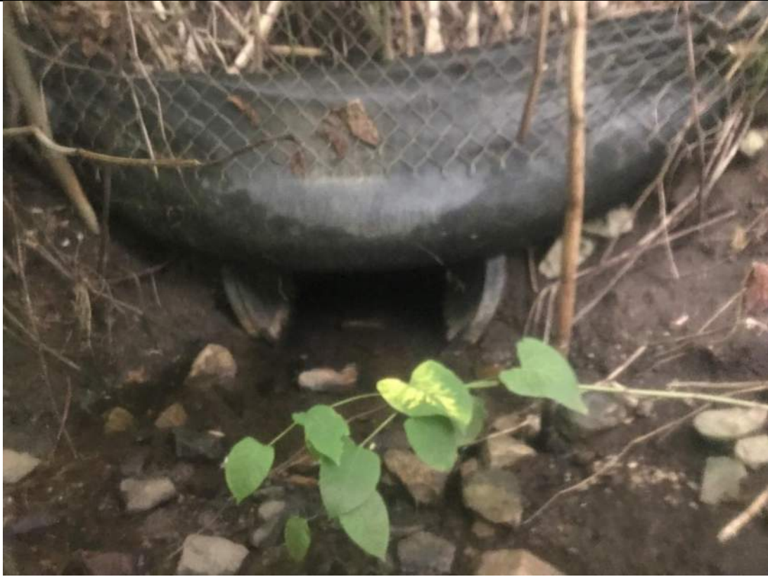
Photograph No. 29 STA 22+25 36"-42" CMP
