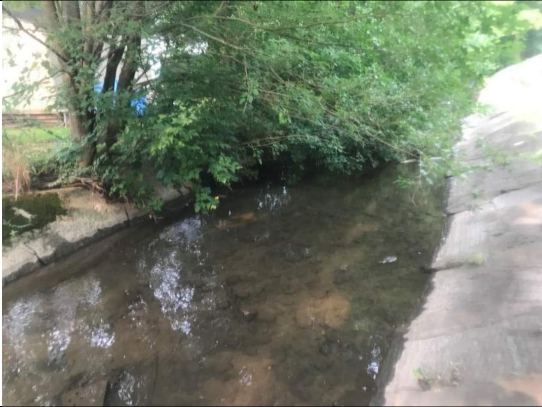
Photograph No. 71 STA 54+00 Downstream photo
