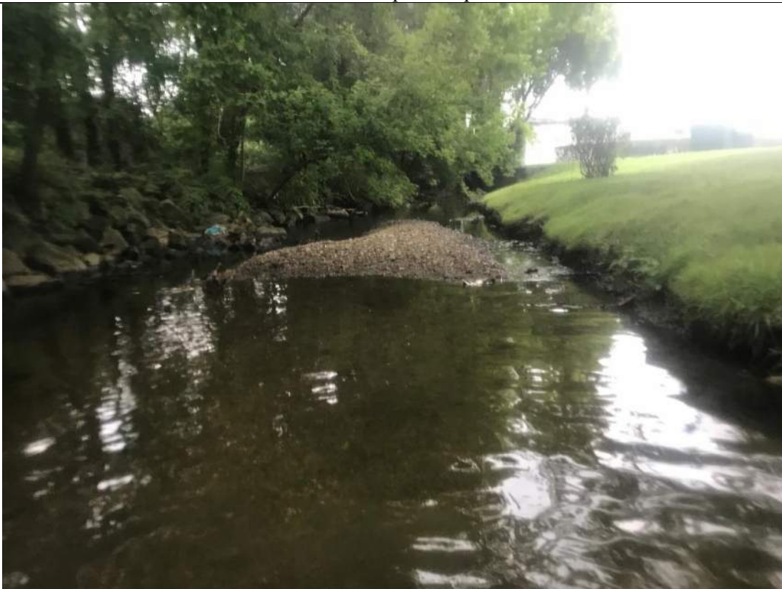
Photograph No. 34 STA 25+50 Downstream photo
