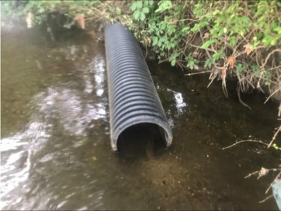
Photograph No. 38 STA 27+00 15" CCP
