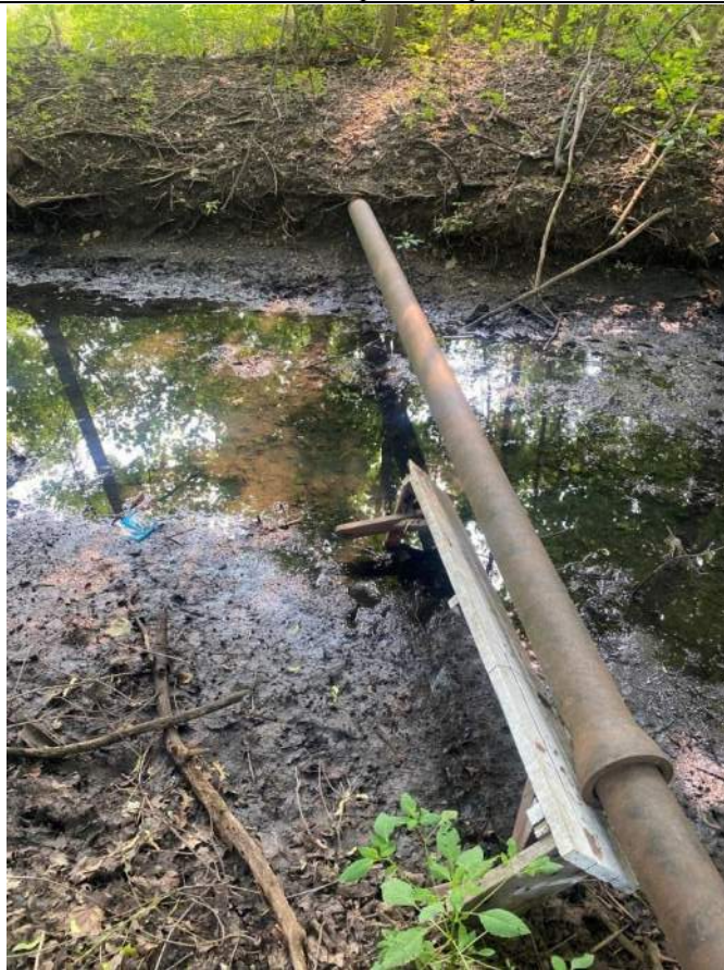
Photograph No. 8 STA 9+50 Pipe crossing
