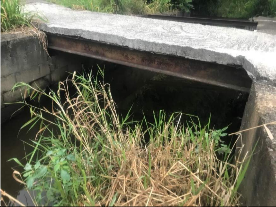
Photograph No. 19 STA 14+75 Downstream photo of bridge
