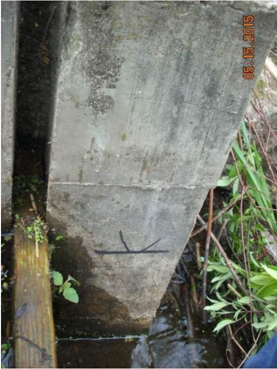
Maximum Lake Elevation marked on west abutment
