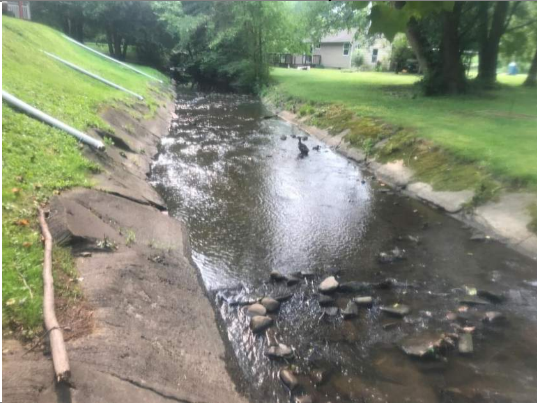
Photograph No. 72 STA 54+00 Upstream photo
