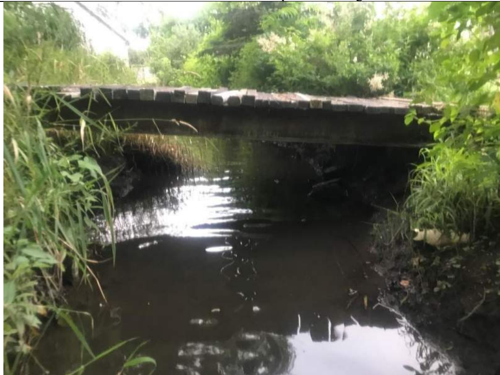
Photograph No. 22 STA 15+50 Upstream photo of bridge
