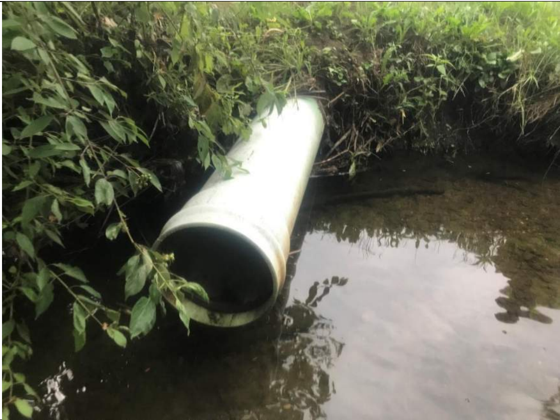
Photograph No. 41 STA 29+50 12" PVC
