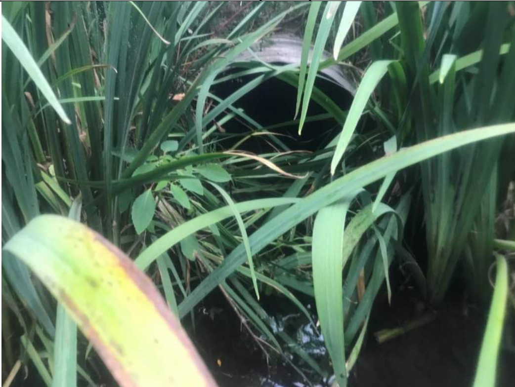
Photograph No. 28 STA 21+25 24" CMP
