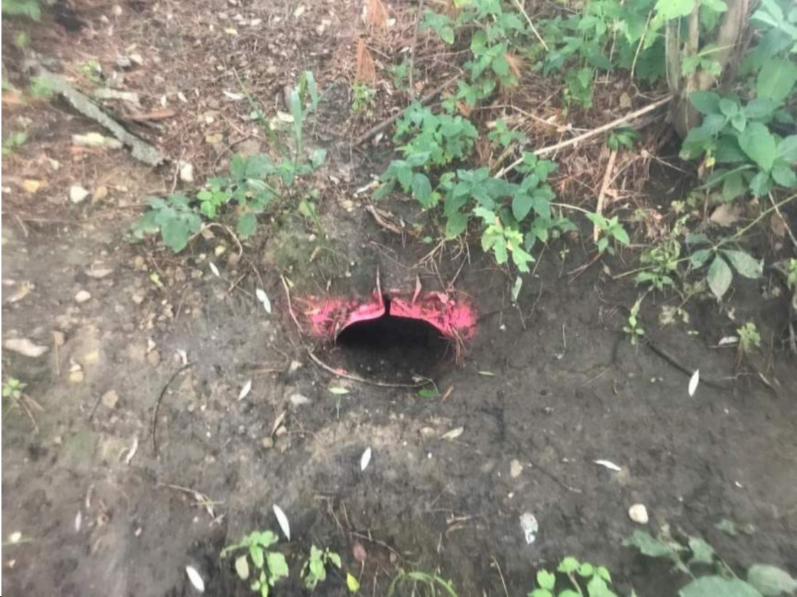
Photograph No. 37 STA 26+50 12" CMP
