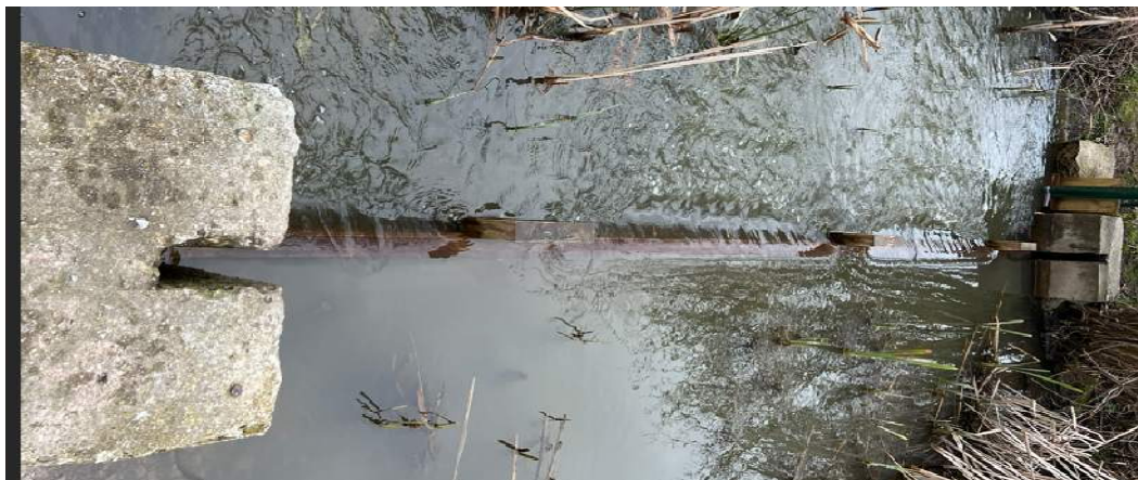
Outfall Structure (East abutment on the left side)
