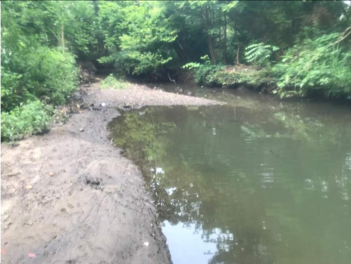
Photograph No. 63 STA 48+50 Downstream photo
