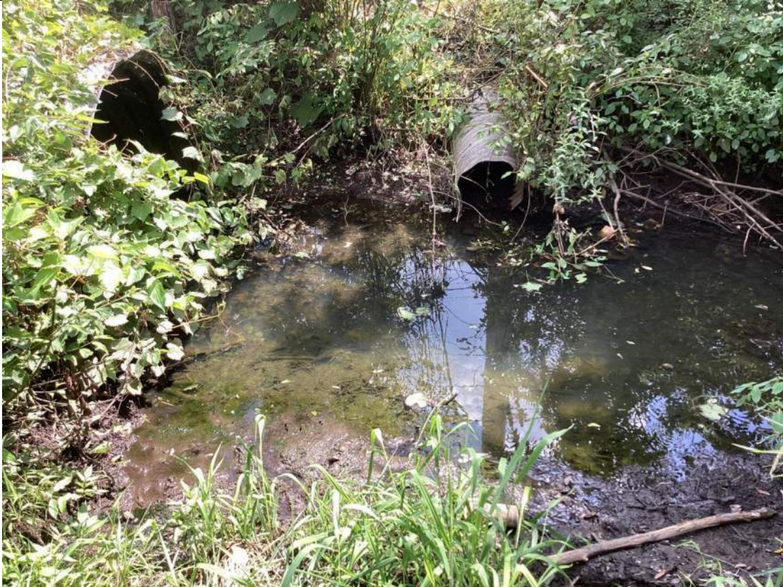
Photograph No. 1 Culverts along Main Channel Stream
