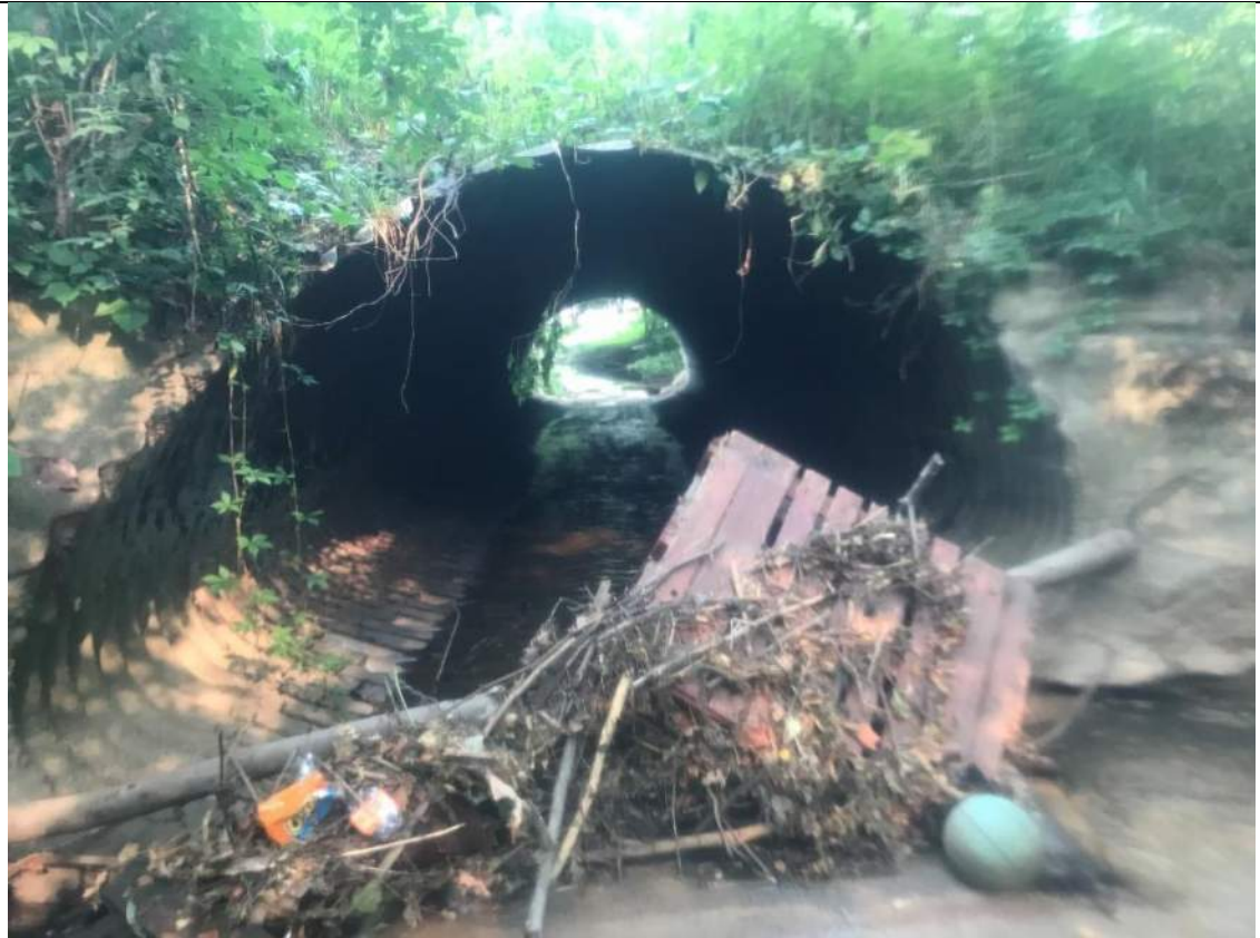
Photograph No. 66 STA 51+00 Downstream photo (11.5ft wide by 7'4" tall road crossing)
