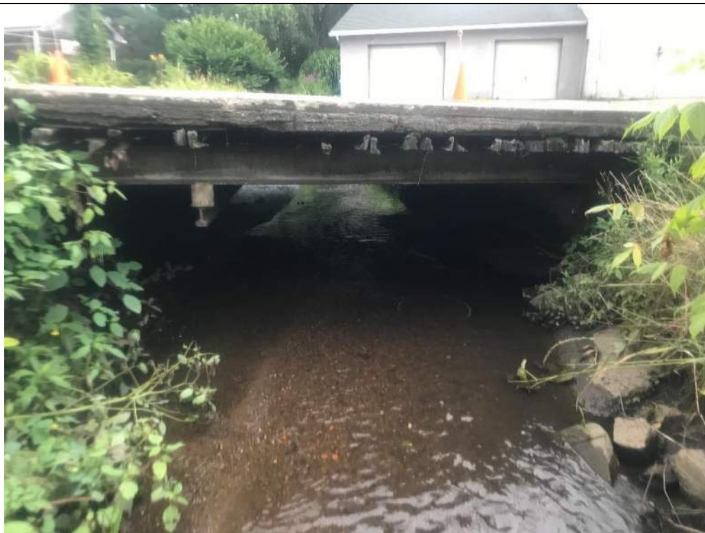
Photograph No. 17 STA 14+00 Downstream photo of bridge (16ft wide by 34" tall)
