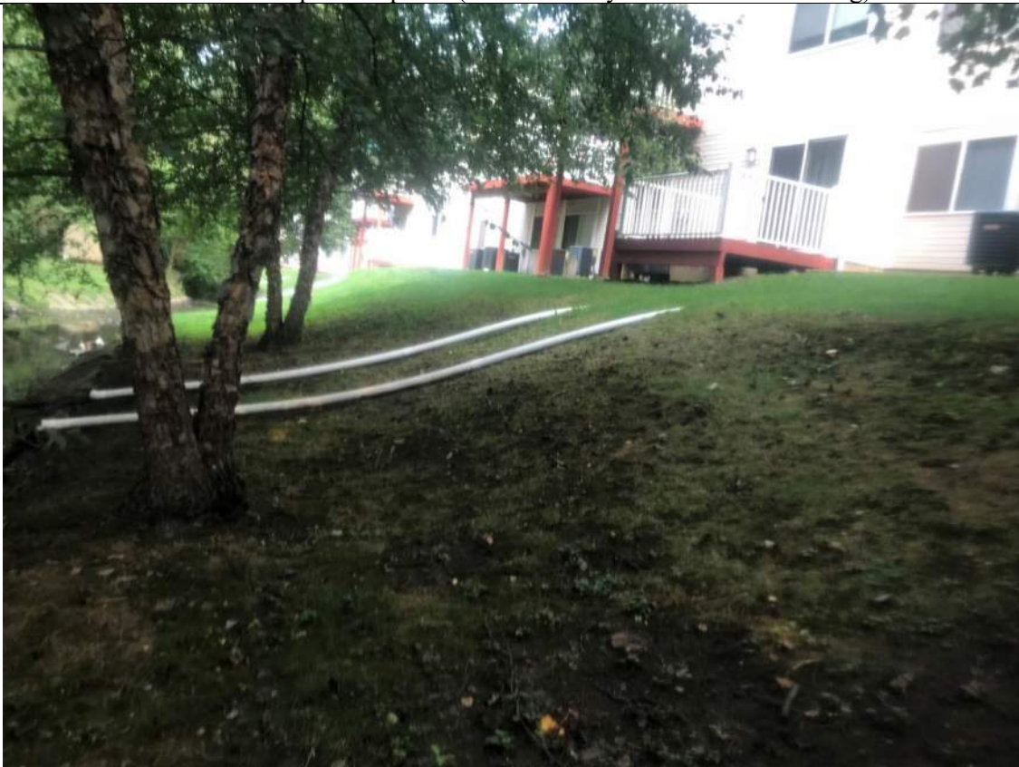
Photograph No. 70 Starting at STA 52+00 downspout outlets run into the creek
