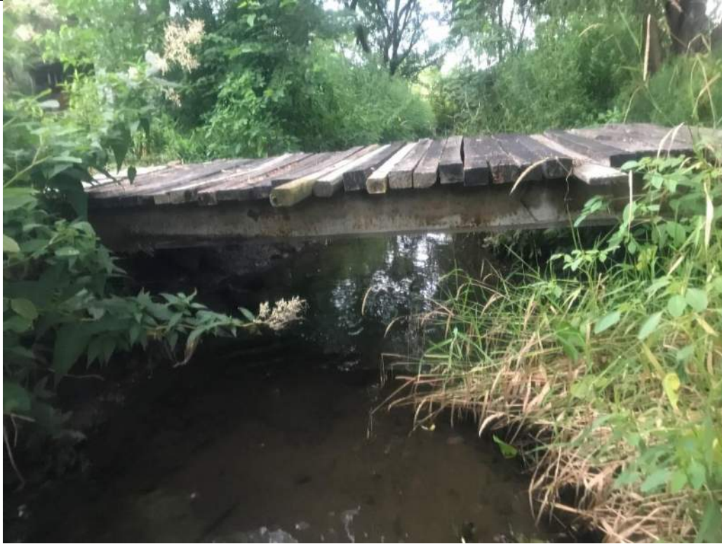
Photograph No. 21 STA 15+50 Downstream photo of bridge
