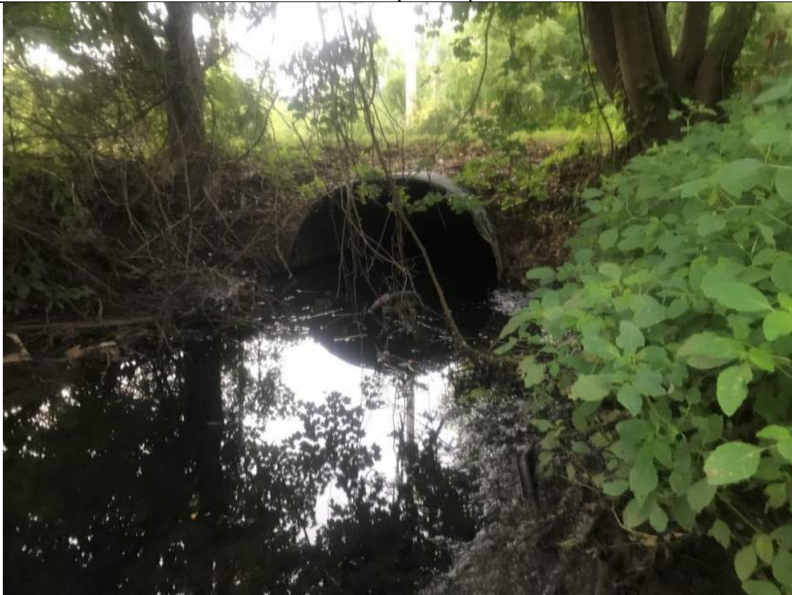
Photograph No. 12 STA 11+00 Downstream photo of 8ft CMP
