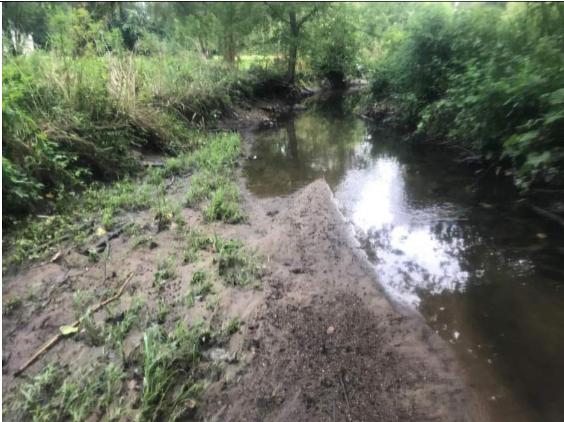
Photograph No. 55 STA 41+00 Downstream photo
