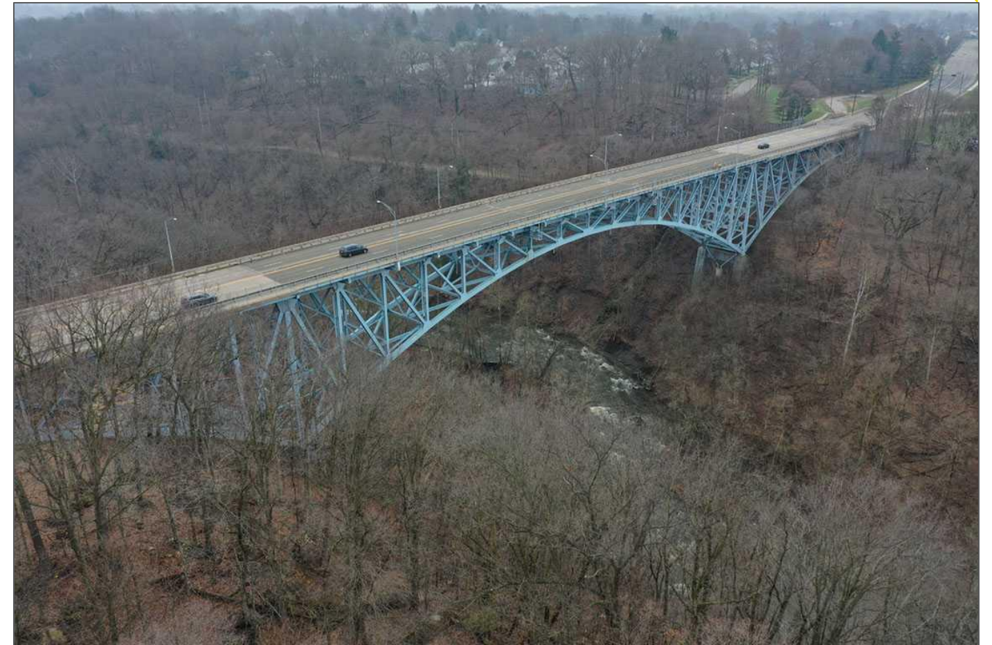
Photo 1: Existing Bridge Elevation Looking Southeast.
