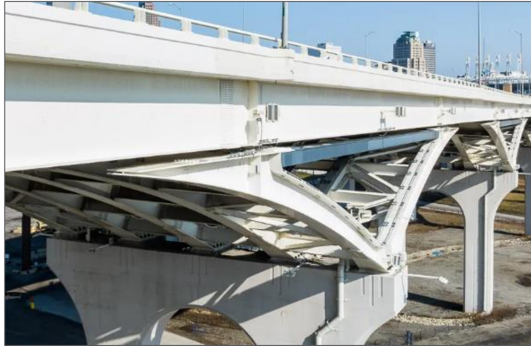
Figure 5: I-90 Innerbelt Bridge, Eastbound Girder Configuration
