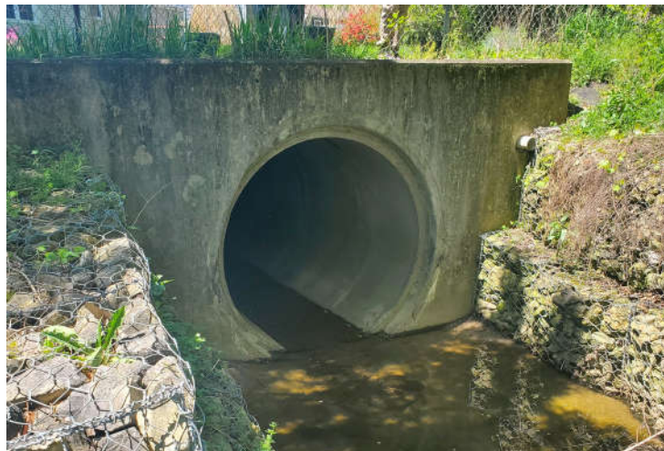
Figure 2.3: Sunnyacres Rd. Culvert, Downstream (72" Rigid Concrete Pipe)
