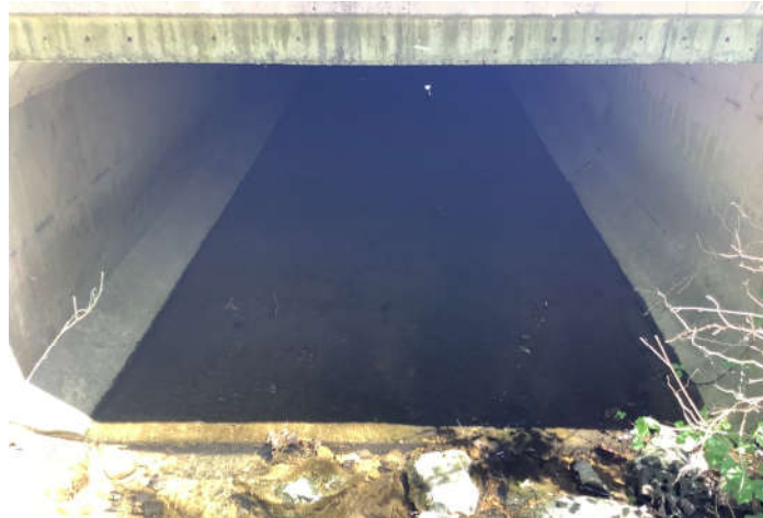
Figure 2.3: Sunnyacres Rd. Culvert, Downstream (72" Rigid Concrete Pipe)
