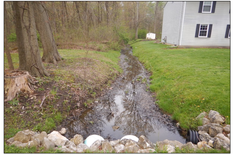
Photo 22: Standing at Marwyck Drive and facing south. Facing downstream of Stream 1.
