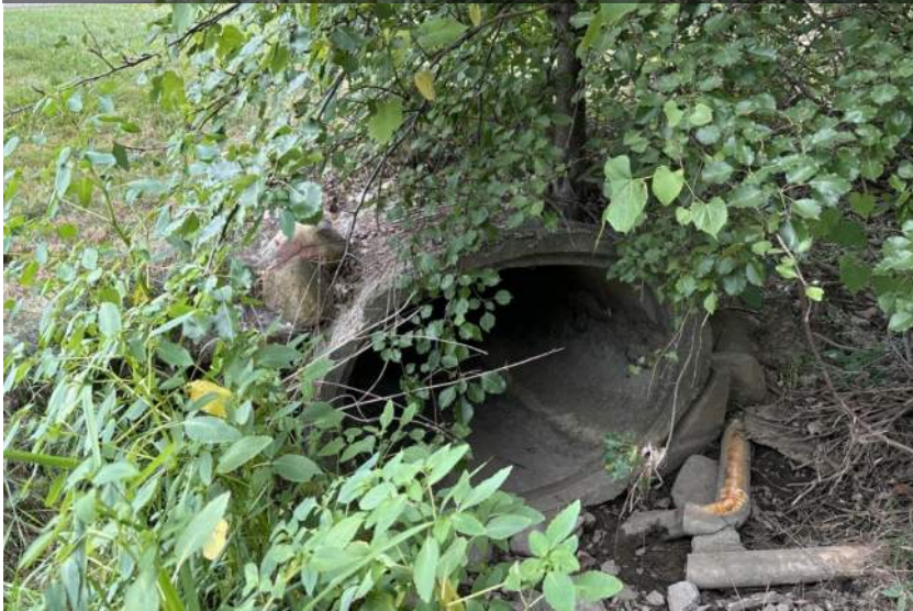
Chaffee Rd Culvert = 53" x 34" (elliptical) U/S end
