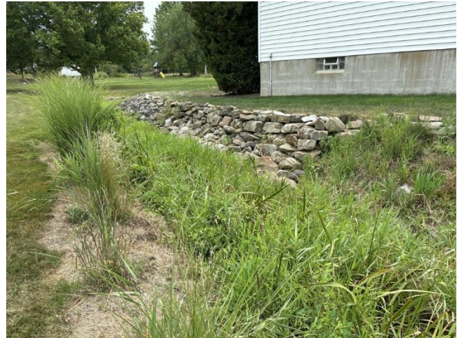
Figure 4. Looking upstream towards channel and corner of 7555 Chaffee Road
