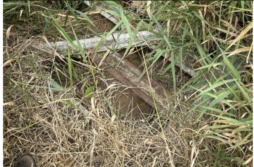
7495 Chaffee Rd culvert (CEI parcel) = 12" D/S end
