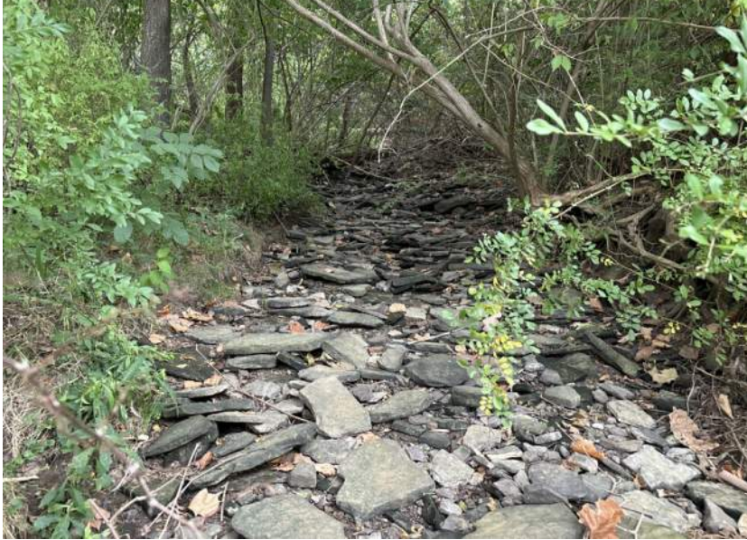
Looking U/S from bike path culvert
