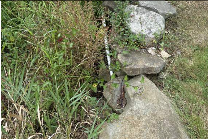
7525 Chaffee Rd backyard culvert = Two 24" D/S end
