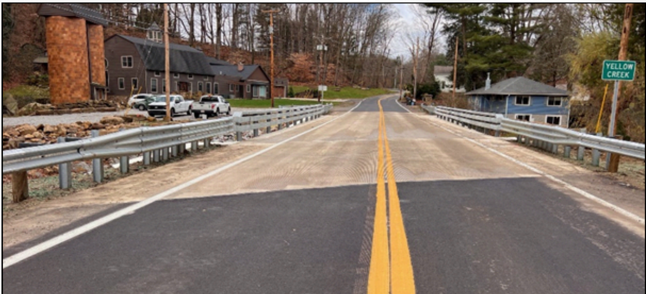
The new Granger Road bridge over Yellow Creek (BAT-079-0221)
