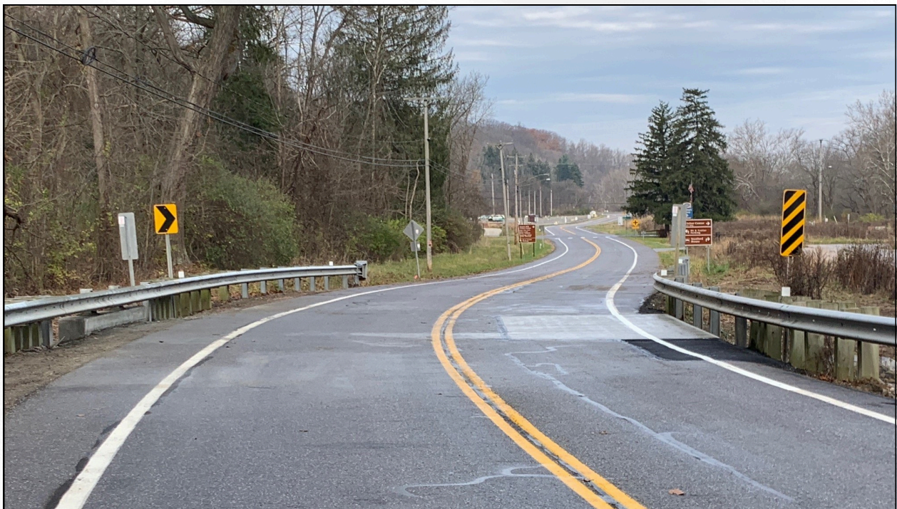
Riverview Rd emergency repair finished work
