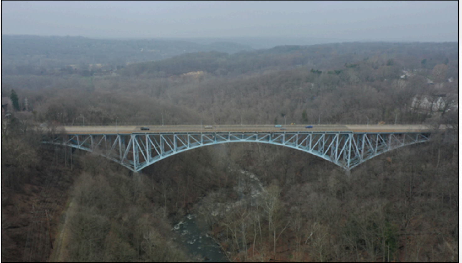
Summit County Engineer's Most Expensive Bridge, The High Level Bridge
