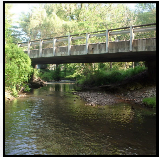
Granger Rd. bridge over Yellow Creek before replacement
