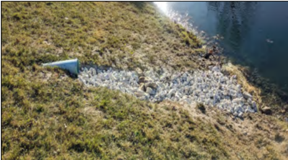
Repaired Erosion at SWMF
