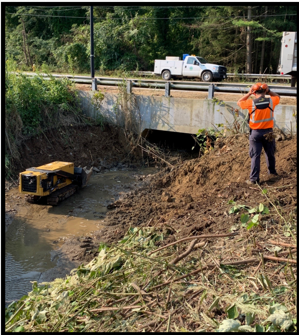
Riverview Rd Bridge (AKR 09-0369)
