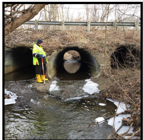
Ira Rd. Bridge over North Fork before replacement
